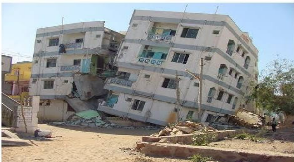
Fig.1. Soft storey building failure during Gujarat Earthquake (2001) in India
